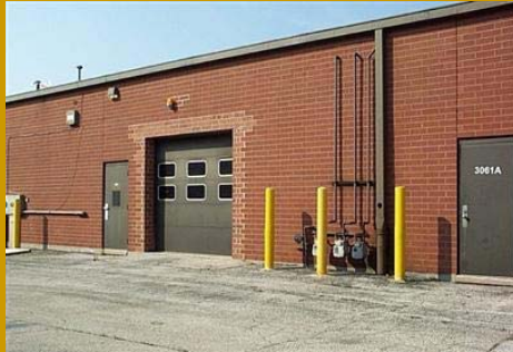
Install roof drains
