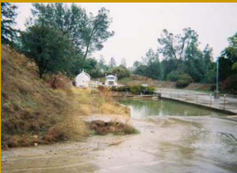
Build settling basin for stormwater and wash water
