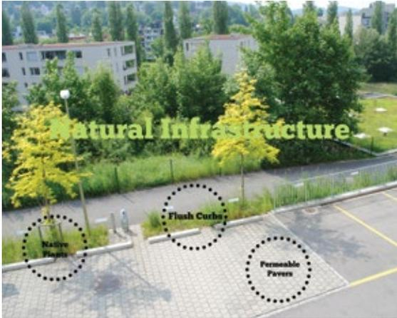
*Low Impact Development features such as permeable paver systems, underground water storage, flush curbs, rain gardens and bioswales can be installed in new development or retrofits can be made to existing infrastructure.*
