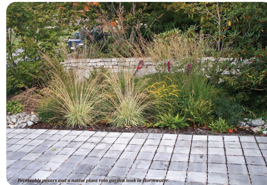
Permeable pavers and a native plant rain garden soak in stormwater.
