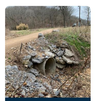
Rain events can cause erosion and weaken unpaved roads, especially around incorrectly sized culverts and clogged culverts. In this photo, the road has narrowed because erosion washed out a six-foot section of colvert.
