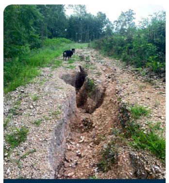
If a road lacks a crown, then potholes and corrugation form because the road cannot properly drain water. Also, weak road base material can contribute to erosion, poor driving conditions, or make the road impassable (as shown in this photo).
