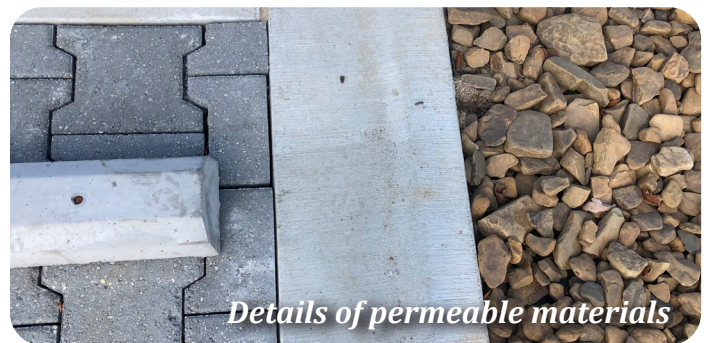
Permeable pavers in parking lot area
