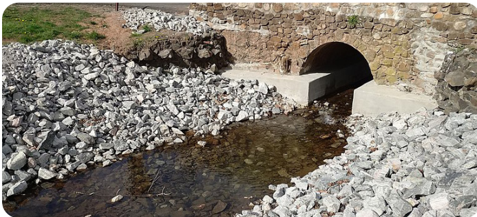
Above: Riprap along a stream. Photo via Wikipedia.
