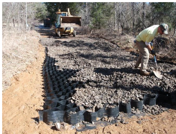
Geocell stream crossing, Lake Wister, OK (Photo: Patterson).
