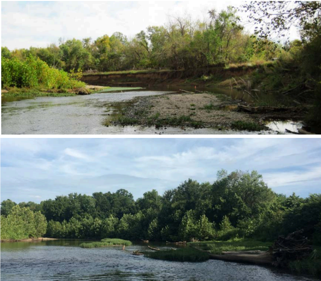
Figure 5-6. Streambank on the White River. Upper shows eroding streambank; Bottom is restored streambank in 2017. Project was constructed in 2012 and protects lands that were historically used for land application of wastewater treatment solids. The project prevents 3,600 tons of sediment and 3,600 pounds of phosphorus from entering the White River and the Beaver Lake watershed, annually.
